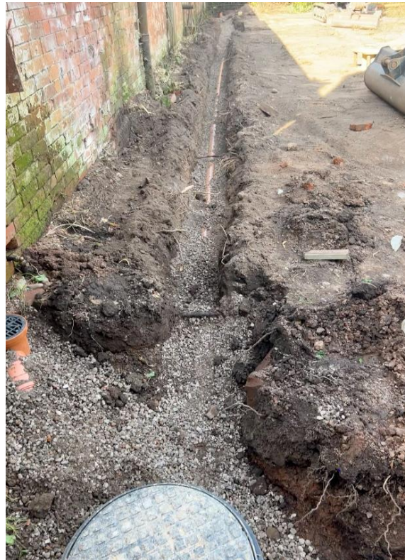
Drainage trenching to the rear of unit 4
