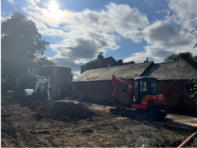
View towards unit 4 and drainage trenching
